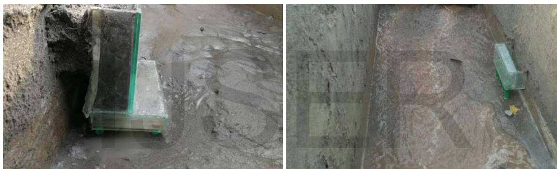
Figure 10: Showing Scour Holes at Wing-wall Abutment of Pushtoon Garhi and at Spill-through Abutment of Haji Bridge
